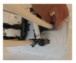
Connections shall be hand tight + 1/4 turn. \*Do not over tighten as stress cracking may result.\*  Connect plumbing line running from (Fresh Tank Out) to "TANK OUT" connection on bottom right of Nautilus panel.
