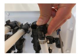
3. On back side of panel, unscrew plumbing line connected to diverter valve end labeled "TO PUMP."
