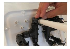
4. On back side of panel, unscrew plumbing line connected to diverter valve end labeled "FROM WATER."
