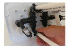
3. On back side of panel, unscrew plumbing line connected to diverter valve end labeled "CITY."
